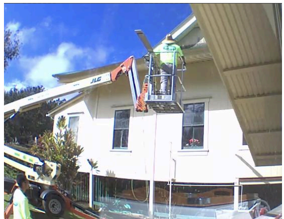
Siding Repair underway in 2023
