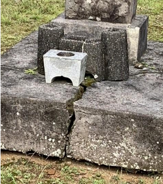
Cracked foundation
