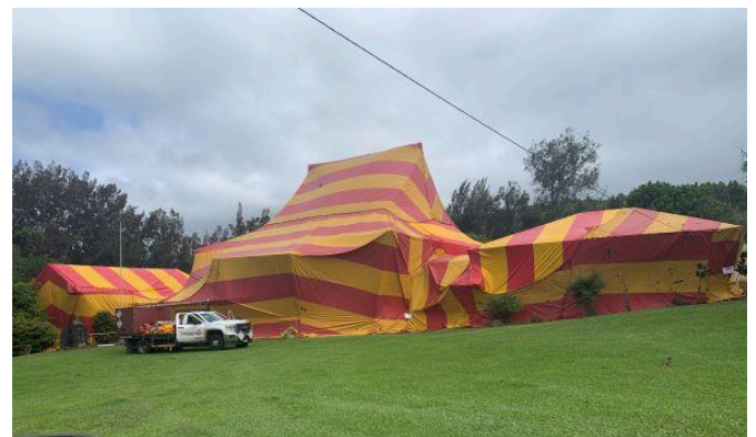
2022 Termite tenting treatment
